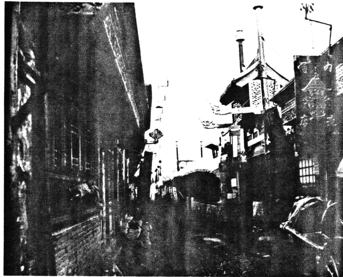
P4-8 AN ALLEY NEAR DASHALA A TYPICAL HUTONG IN A COMMERCIAL AREA
