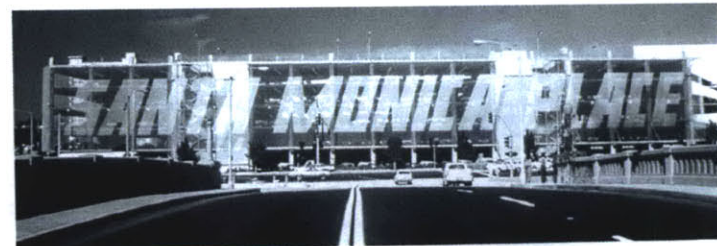
"Sign" skin: FIG. 01-34 literally tells the type of space (Frank Gehry, chain link veils for the parking structure at Santa Monica Place)
