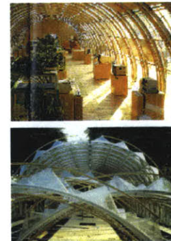
FIG. 01-21, 22 The IBM Travelling Pavilion by Renzo Piano is portable building. The load-bearing frame consists of glu-lam arches with the intermittent spaces between the arches being transparent sheets of polycarbonate. In its unaffected simplicity the refined and repetitive series forms a rich pattern..
