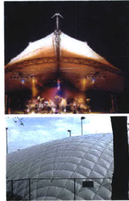
FIG. 01-14, 15 Temporary performance spaces created with tensile and pneumatic structures
