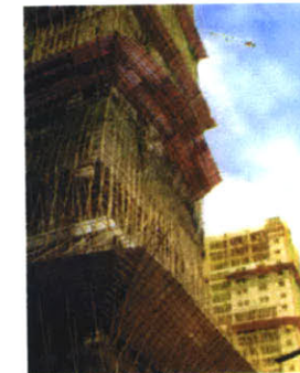
(top two) FIG. 05-01, 02: high & low tech connections (bottom two) FIG. 05-03, 04: structural lattice formed by bamboo
