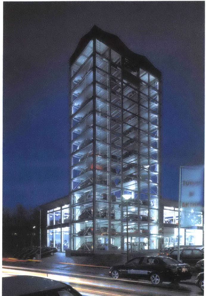
Recently, automated parking structures are now employed to utilize extremely tight sites as well as to make spectacle of the parking process as with this car tower for a toyota car dealership.
