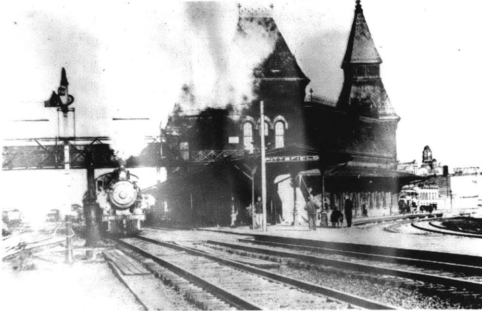
First generation rail station 1865-1890. Courtesy of the Berkshire Athenaeum, Pittsfield, Massachusetts.
