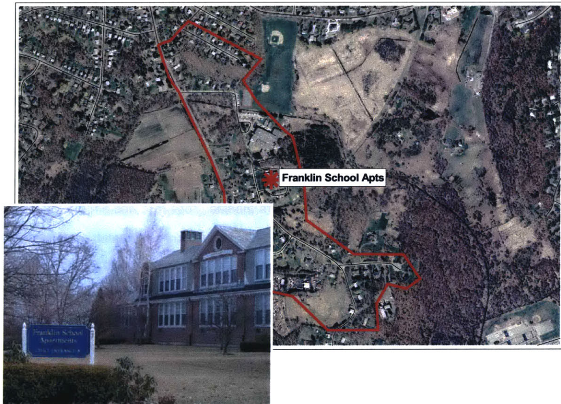
Figures 7.28, 7.29 Franklin School Apts Aerial and Site Photographs
