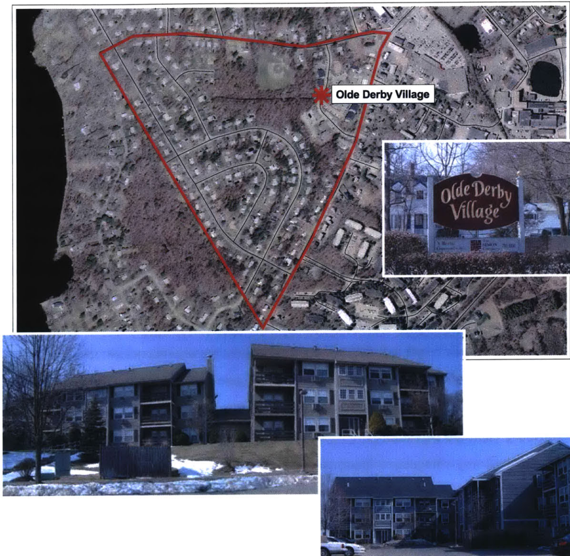
Figures 7.5 - 7.8 Olde Derby Village Aerial and Site Photographs
