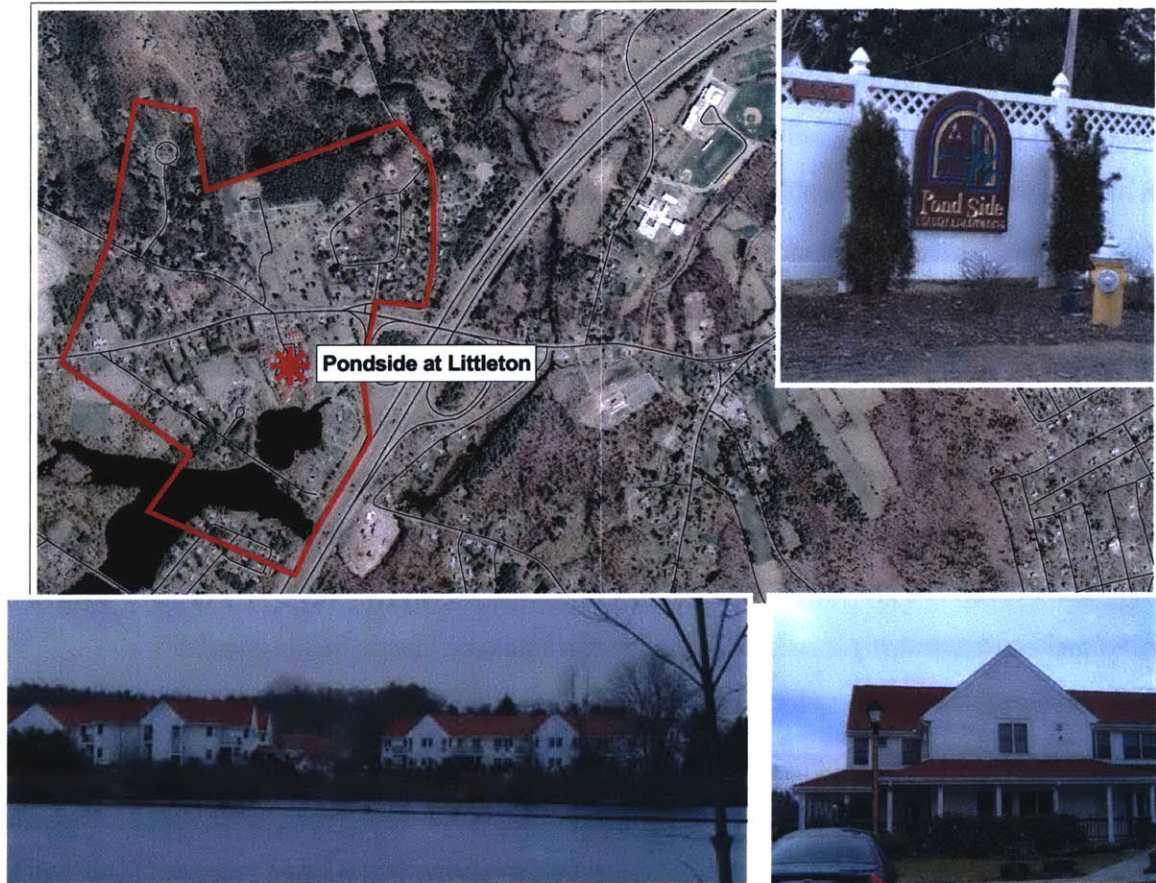
Figures 7.17 - 7.20 Pondsides Aerial and Site Photographs
