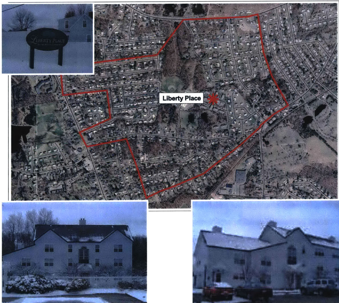
Figures 7.24 - 7.27 Liberty Place Aerial and Site Photographs
