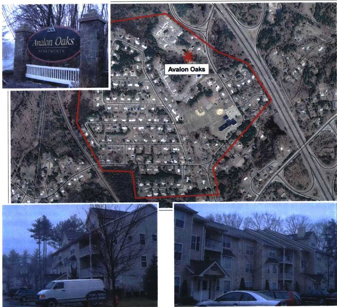
Figures 7.9 - 7.12 Avalon Oaks Aerial and Site Photographs
