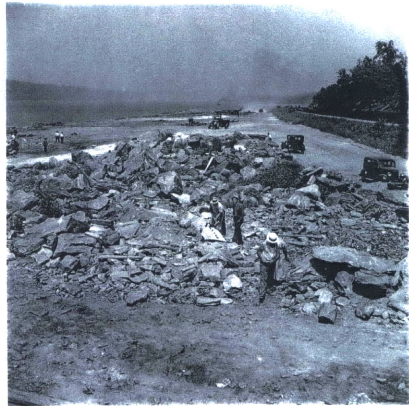
Westside improvement, north of Dyckman St. 8/13/1936
