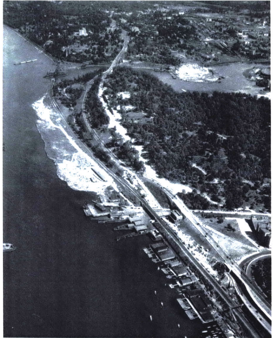
Aerial view of site from the south. 9/8/1937
