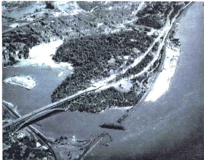
Aerial view of site from the north. 6/25/1938
