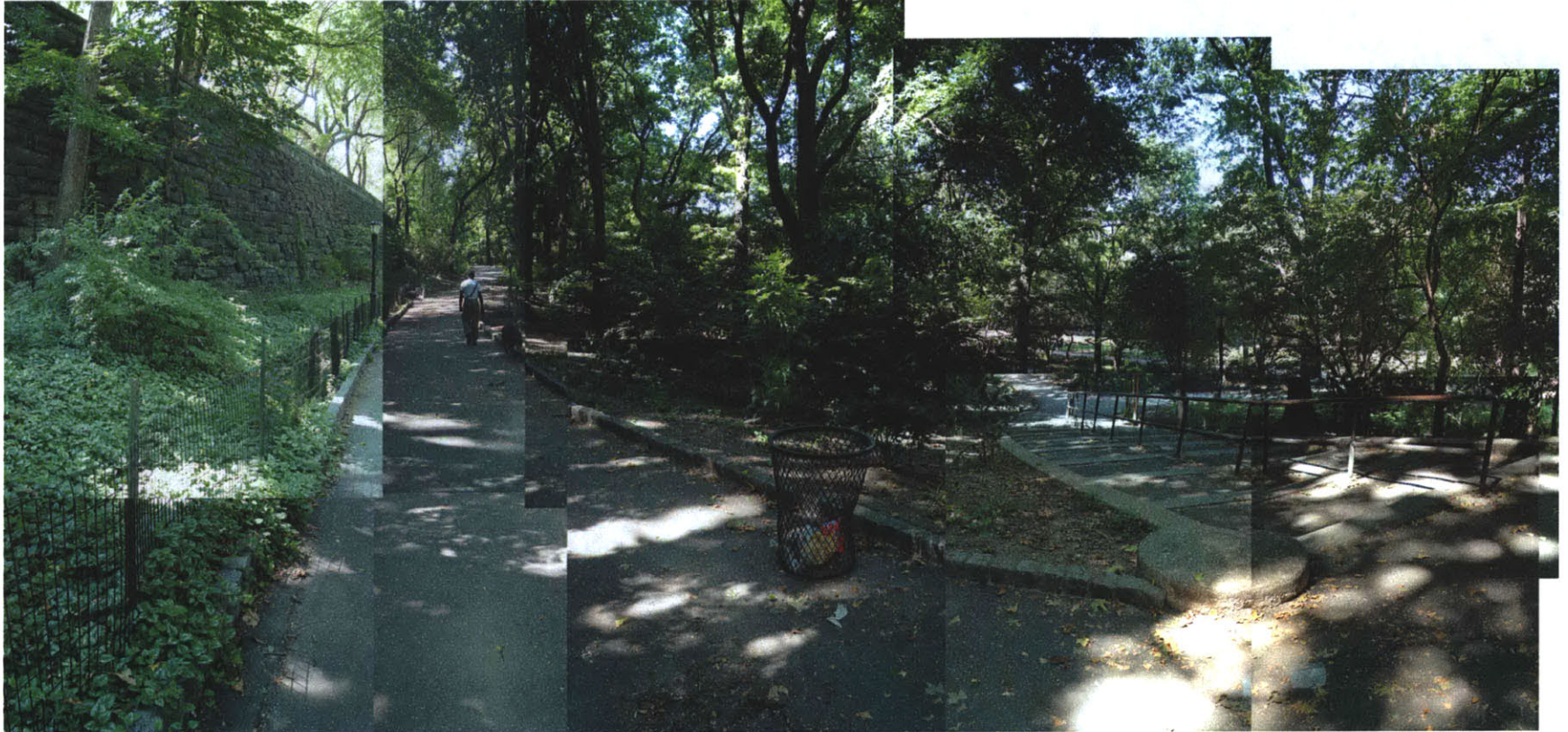
fig 29: the retaining wall on the left runs from 98th to 120th.
