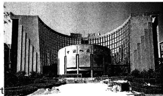
Fig 4.3: The Bank of China (above) and the People's Bank of China (below)
