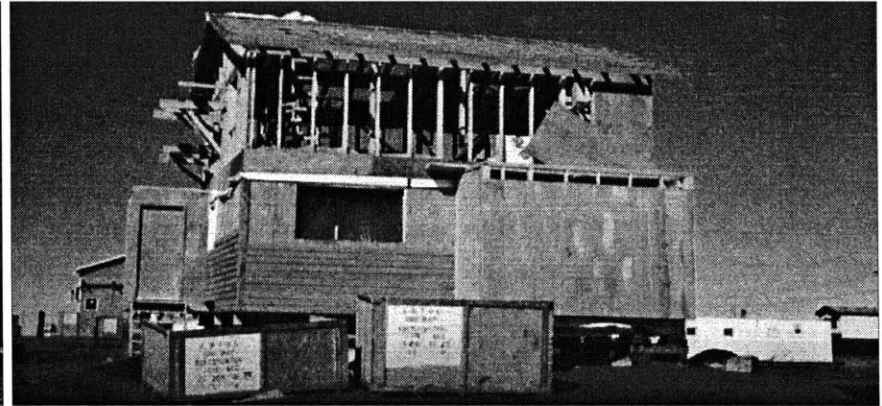
Fig 1.2.2 HAP house construction
