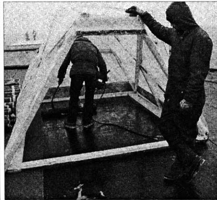
Fig 3.1.2 Roofing in Rankin Inlet, October
