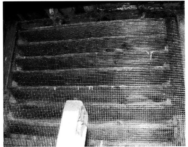
Figure 4-22 Left : View looking up into cupola after paneling was removed: three interior faces. Right : Unobstructed interior face of one side of the cupola, showing the 1/2” screen.
