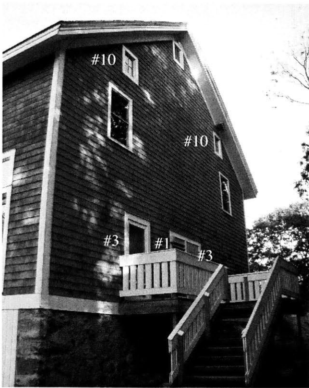
Figure 4-4 Rear (East) of building, showing operable Attic 2 windows (#10), Conference and Assembly room doors (#3), and the East louvered door (#1). The unlabeled windows (two larger Attic 1 windows and one small Attic 2 window) are not operable.
