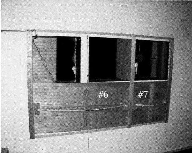
Figure 4-15 Retrofitted apertures to the Attic, with sliding covers. View from below with both sliders open and closed. Left : Note the compartment made to isolate the fan from the rest of the opening (to prevent backflow of Attic air). The large slider covers the pre-existing aperture (at left) and a portion of the opening created by the removal of the stairs.
