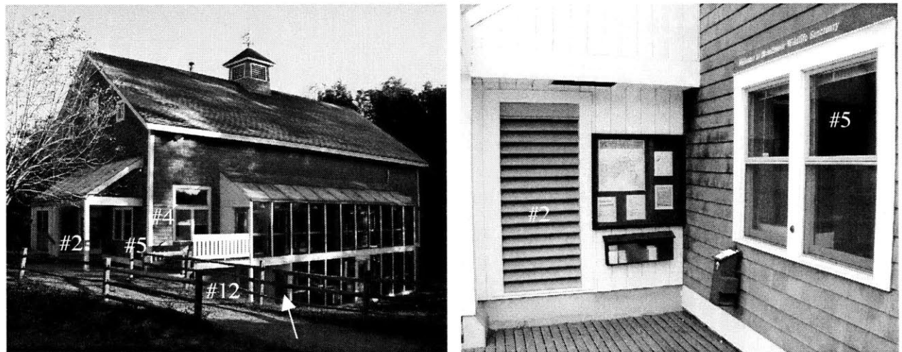
Figure 4-2 Left : View of building from Southwest. Note aperture #2 on the wall perpendicular to the front door. The white arrow shows the louvered door kept open all summer to vent hot air from the Sunspace. Right : View of the louvered door to the right of the main entrance.
