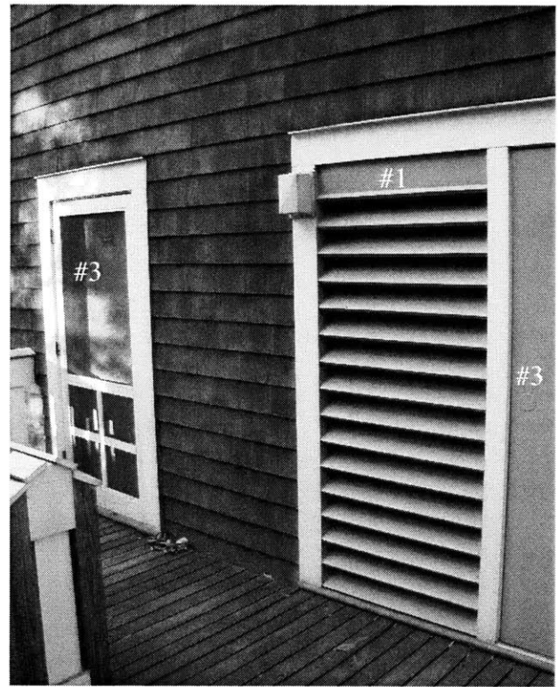
Figure 4-4 Rear (East) of building, showing operable Attic 2 windows (#10), Conference and Assembly room doors (#3), and the East louvered door (#1). The unlabeled windows (two larger Attic 1 windows and one small Attic 2 window) are not operable.
