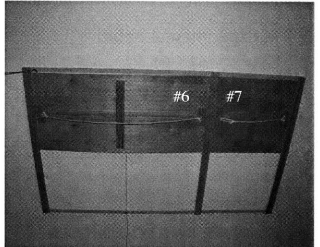
Figure 4-15 Retrofitted apertures to the Attic, with sliding covers. View from below with both sliders open and closed. Left : Note the compartment made to isolate the fan from the rest of the opening (to prevent backflow of Attic air). The large slider covers the pre-existing aperture (at left) and a portion of the opening created by the removal of the stairs.
