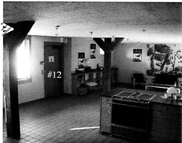
Figure 4-13 Common Room in Basement. Note Basement Door (#12) and Basement thermocouple location (9).
