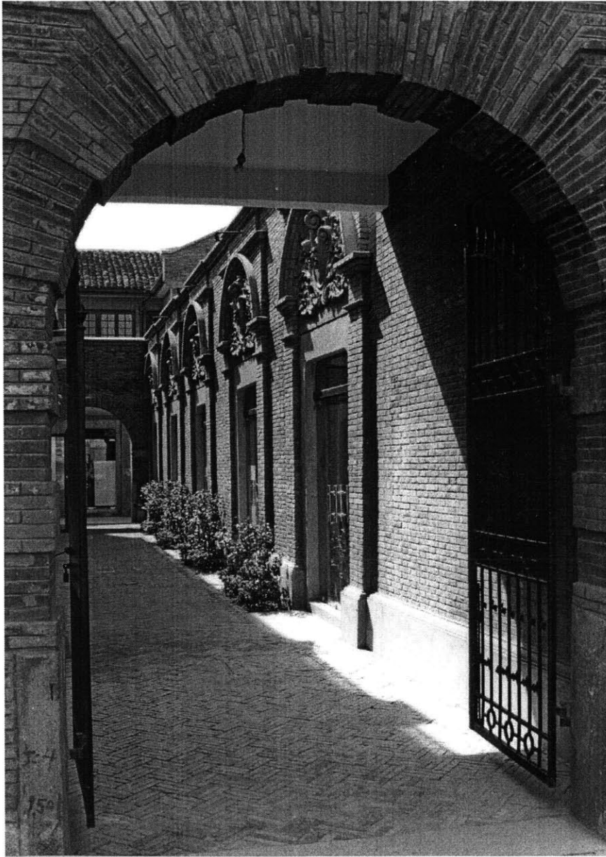
Figure 4-6. The Preserved Street Patterns and the Exterior of the Shikumen Buildings
