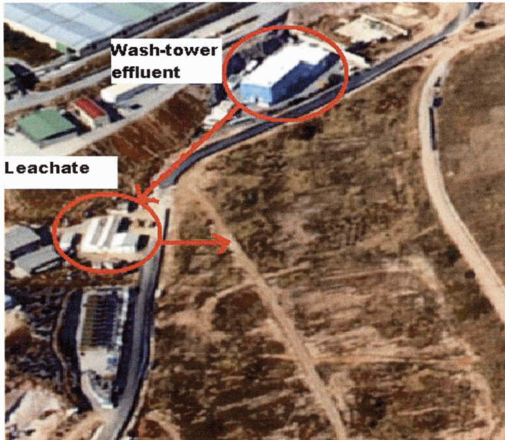
Figure 11: Incinerator to Leachate facility
