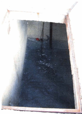
Figure 3: Final Product of Leachate Treatment System
