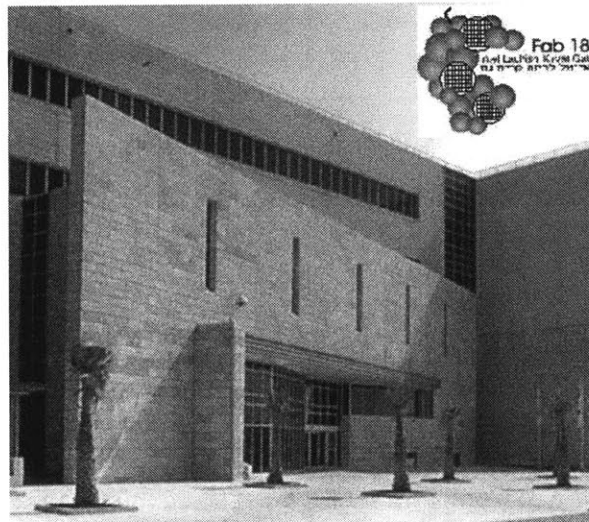
Figure 4: The front entrance to Fab 18 in Qiryat Gat, Israel
