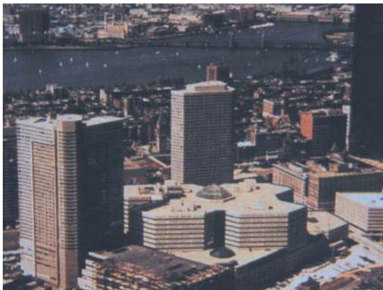
Copley Place completed development
