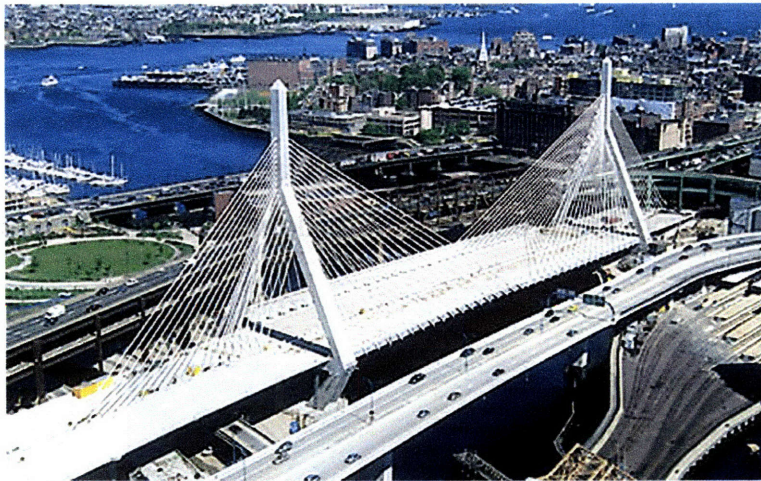
Image 3.1 The cable-stayed bridge over Charles River in Boston, MA 2
