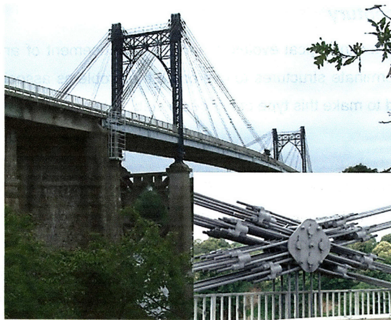
Image 2.8 Lezardrieux Bridge completed in 1925 7
