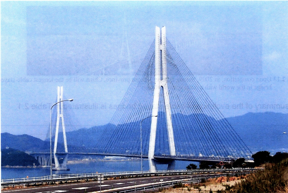
Image 2.12 Tataru bridge, Japan is currently the longest cable-stayed bridge in the world with a main span of 890m 11
