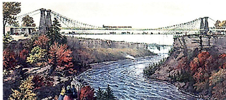
Image 2.4 Niagara Falls Railroad Bridge completed in 1855 3
