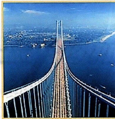
Image 1.4 Akashi Kaikyo suspension bridge in Japan with a single span of 1,991 meters 4
