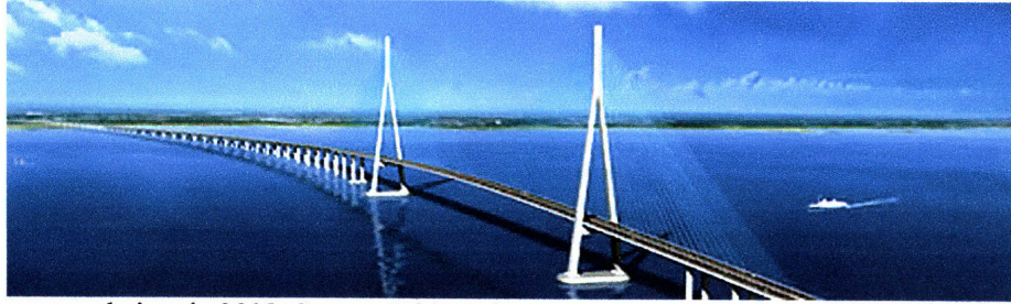
Image 2.13 Upon completion, in 2009, Sutong Bridge, Jiangsu province, China will be the longest cable-stayed bridge in the world with a main span of 1088m 12
