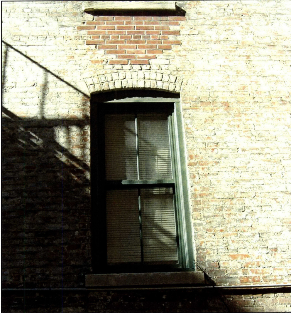
An apartment window facing the lightwell
