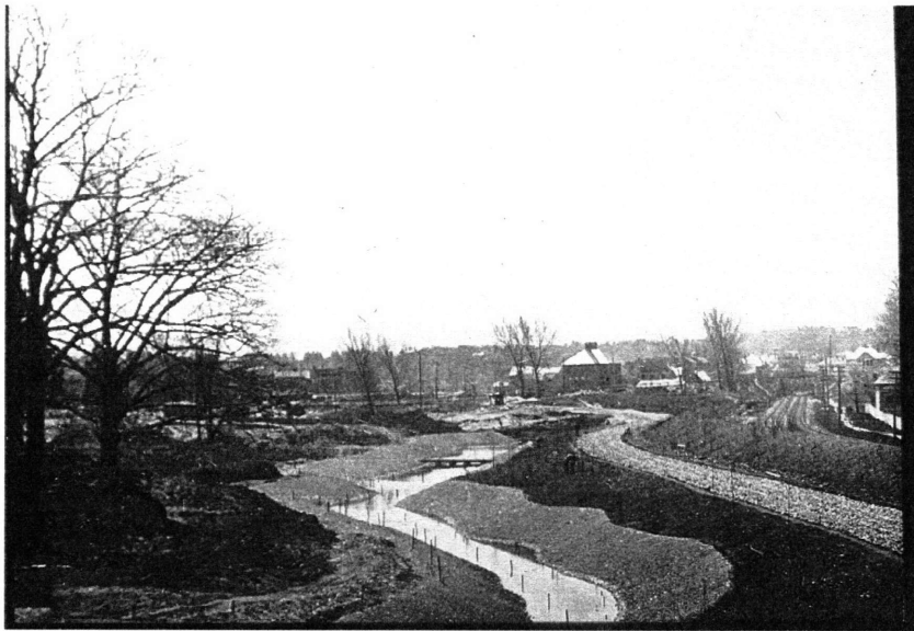
Grading and fortification of river embankment, Muddy River. (Courtesy of the Loeb Library, Harvard)
