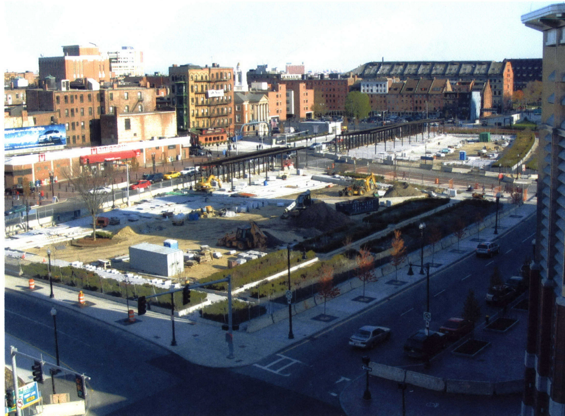
VIEW OF GREENWAY FROM LIBRARY
