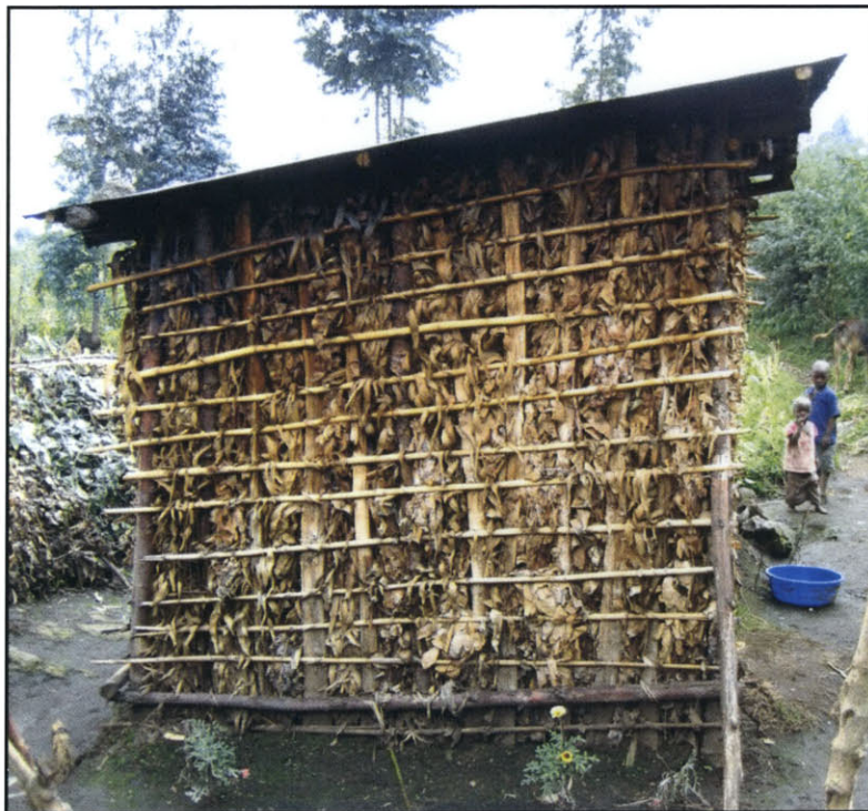
Figure 38: Poor-level house with branch walls in Bisate Village (Picture by Author)
