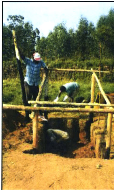
Figure 57: Building the frame (Rees 2000)
