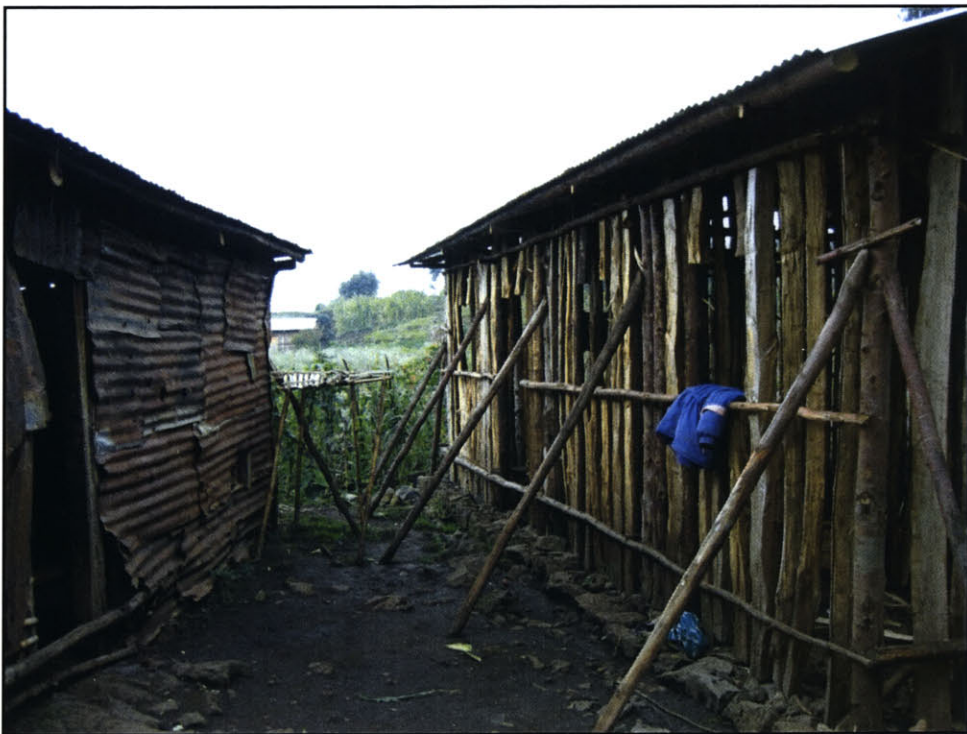
Figure 40: Higher-level house in Bisate Village (Picture by Author)
