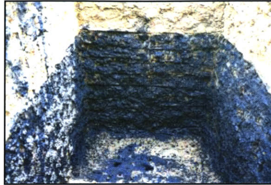
Figure 56: Coating the cistern's walls with old engine oil (Rees 2000)
