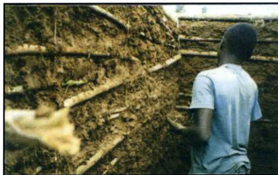
Figure 59: Illustration of plastering walls with mud (Rees 2000)
