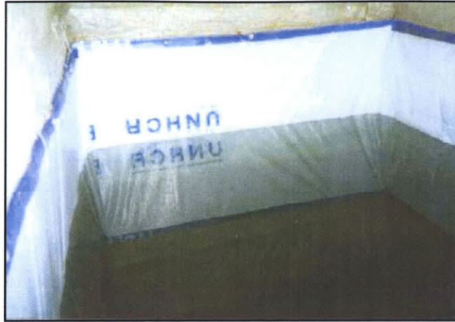
Figure 60: Lining the cistern with tarpaulin sheet (Rees 2000)
