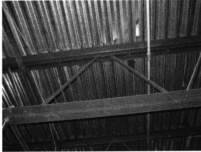
Figure 4-5: Steel Joist and Metal Deck (Homem)
