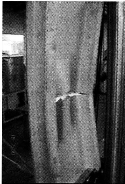
Figure 3-62: Final deformed shape of the TSCCT specimen
