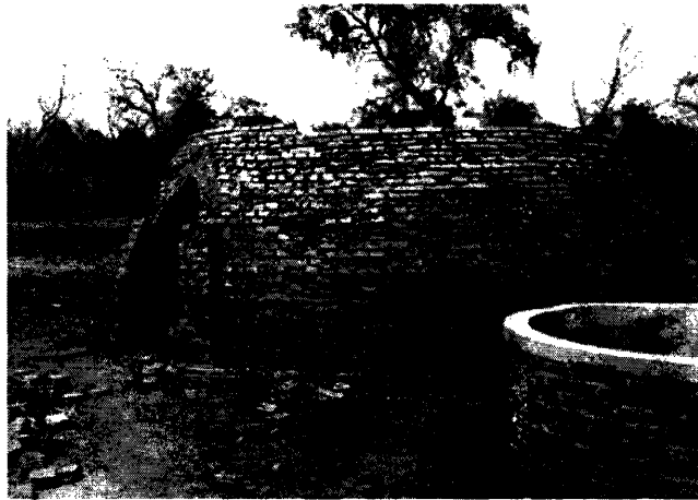
Figure 6. Argentine Half-Orange Kiln
