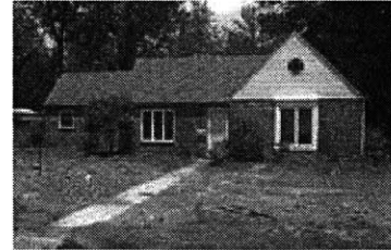
Figure 3: Home in Hollin Hall Ready for Demolition
