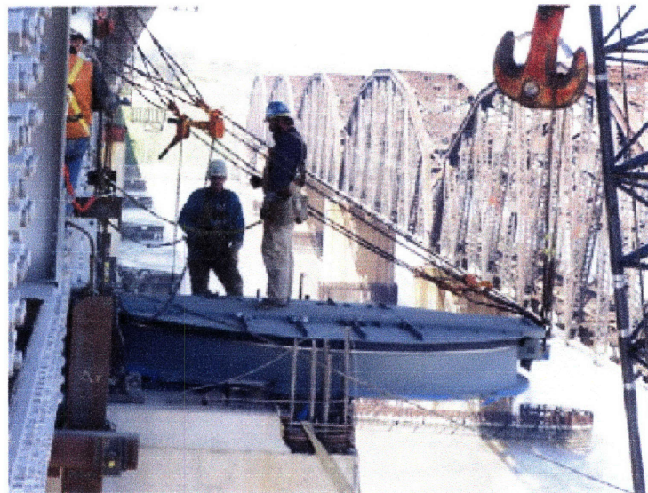
Figure 52: Inverted pendulum being installed on the Benicia-Martinez Bridge in California (Roberts, 2005)
