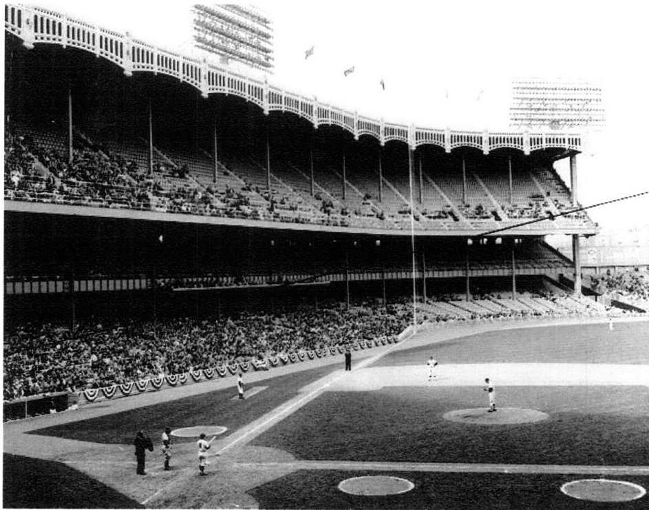
Figure 5-14: Left field at Yankee Stadium featuring the trademark façade [3]
