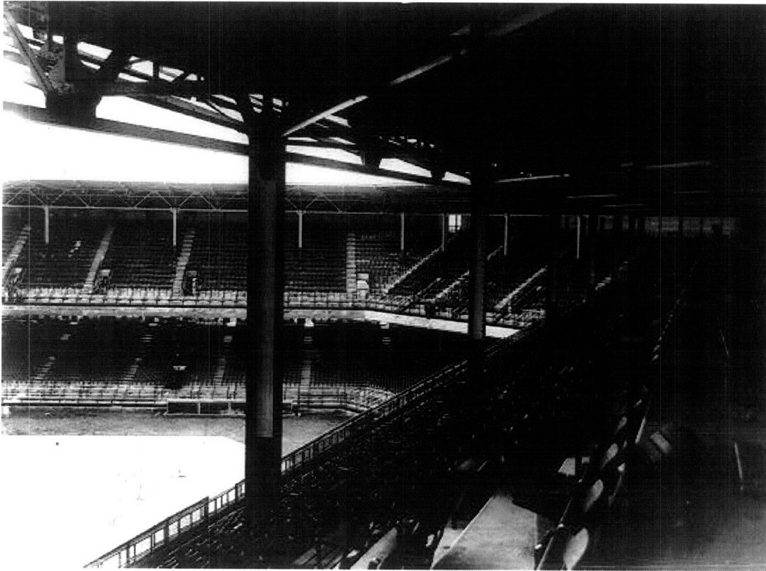
Figure 5-8: Steel supports at Ebbets Field [3]
