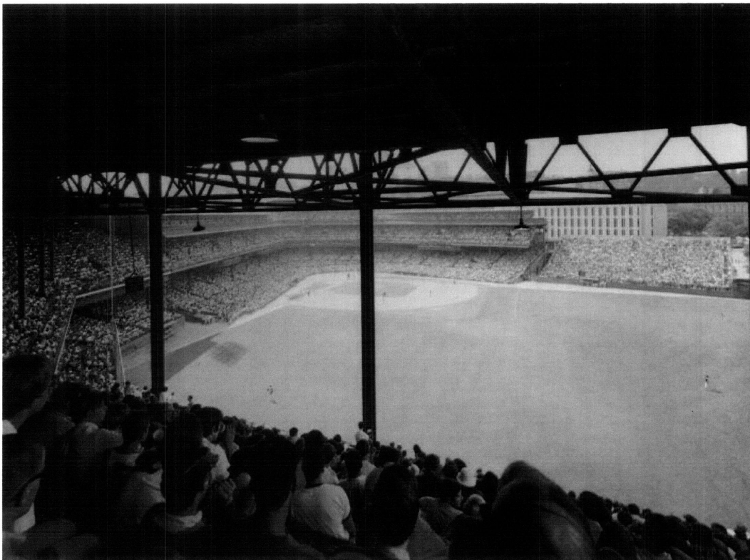
Figure 5-2: Steel columns and trusses supporting roof at Forbes Field [3]
