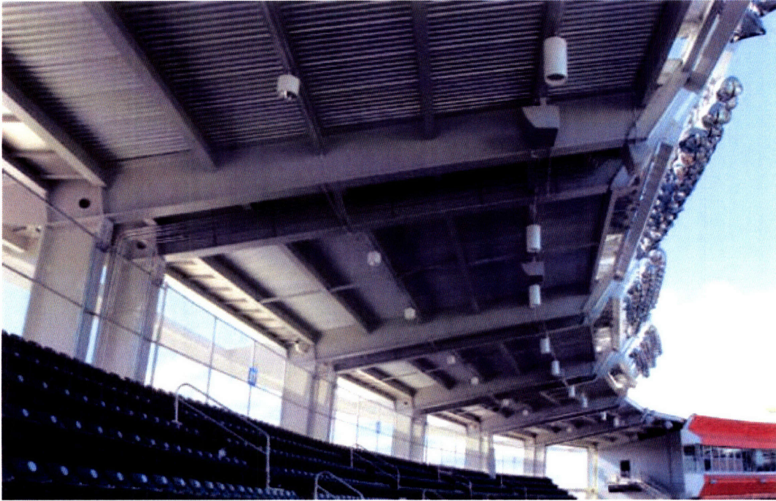
Figure 8-4: Cantilevered roof at Nationals Park [10]
