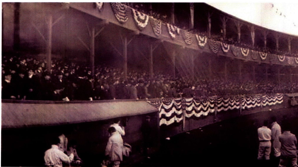
Figure 4-2: Grandstands at the Polo Grounds [3]
