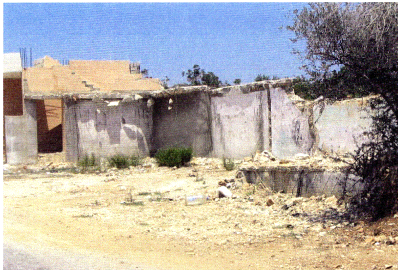
Figure 17. House destroyed during the July 2006 war. The underground cement reservoir for rainwater is still visible on the right
