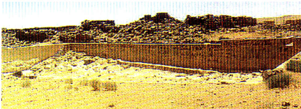
Figure 16. A birki for community rainwater collection (Oweis et al., 2004).
