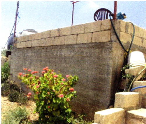
Figure 9. Above ground cement cistern.
