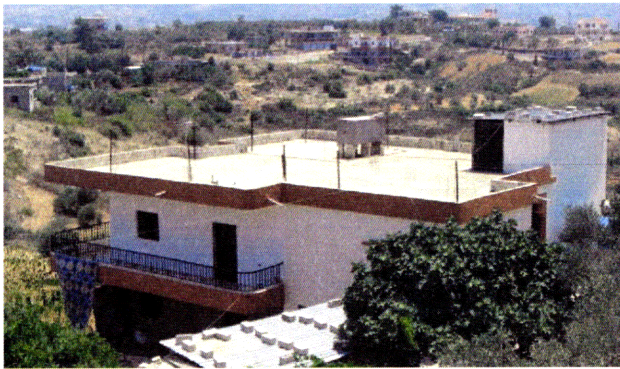
Figure 7. Typical cement rainwater-collecting rooftop.
