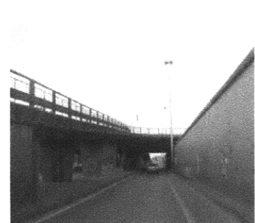
Figure 1.27: Ramp leading to the Seaside Road.
