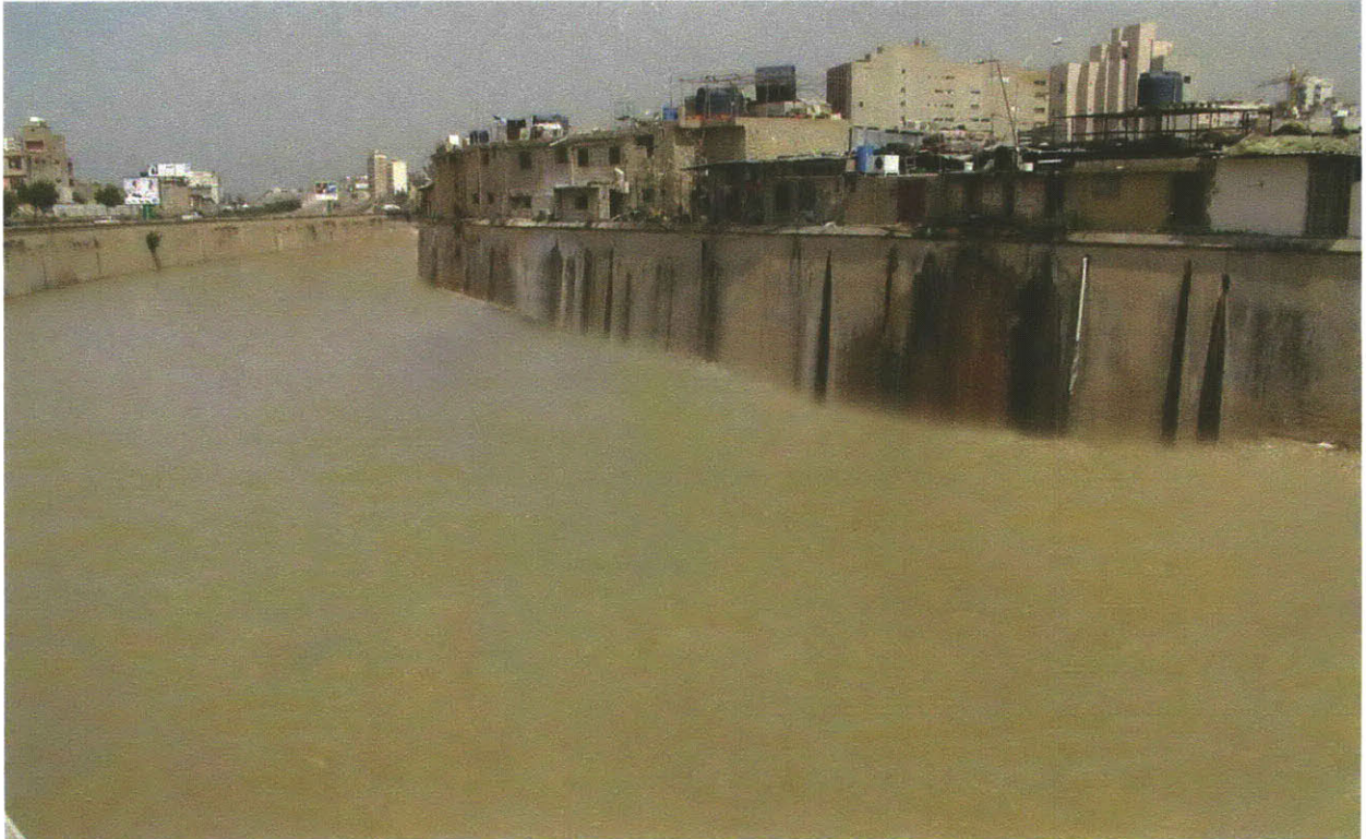
Figure 3.21: Wet season Condition
