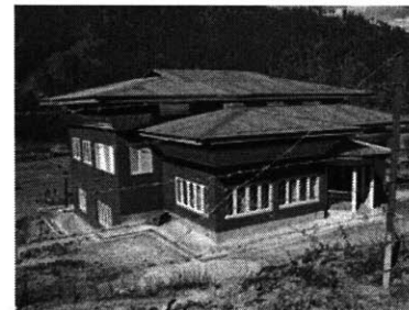
New houses as shown in these images are most often painted reinforced concrete. When brick is used, it is usually covered from sight. Very few local traditional materials are used.
