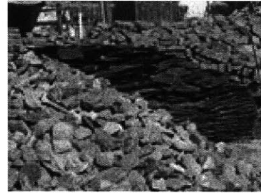
Quality materials of stone, slate, and brick (as shown above) are used less frequently than reinforced concrete.
