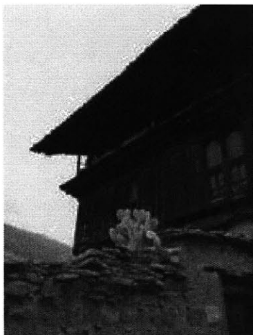
These traditional farmhouses are constructed of rammed earth with timber substructure for the upper floors.
