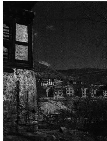
The traditional rammed earth farmhouse in the foreground is surrounded by the new reinforced concrete structures.
