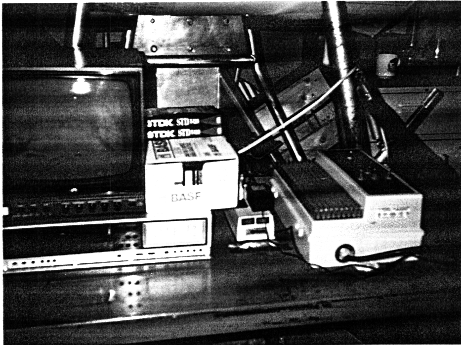
Figure 3-7 Video Monitoring/Recording System
