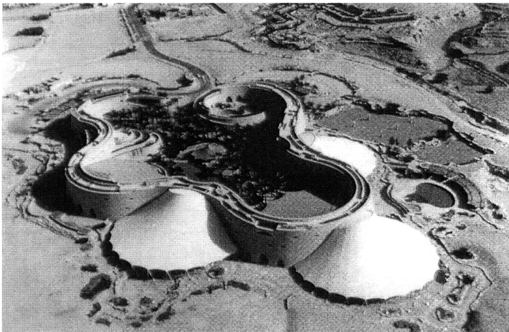
Figure 1.6 Masonry construction in combination with structural membranes and cable-nets, built to house the Diplomatic Club in Riyadh.
