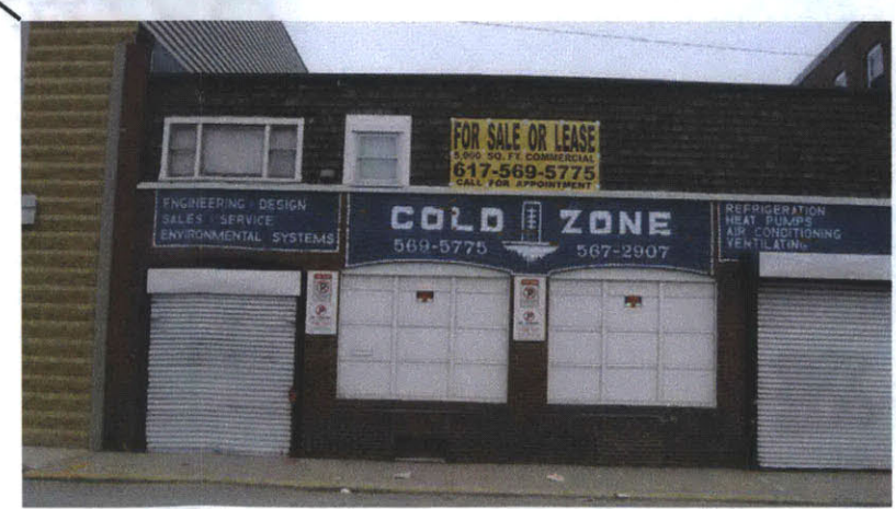
Several unused-looking buildings along this block.
