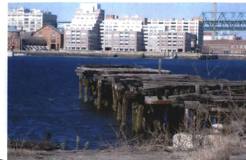
View of Charlestown waterfront from site.
