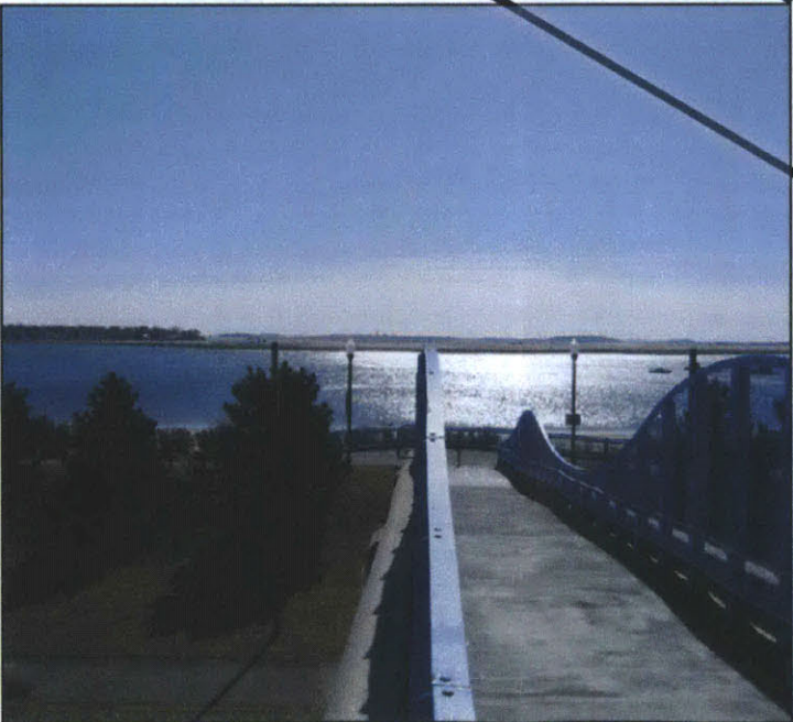
A pedestrian bridge recently built between Bennington St. and the beach.
