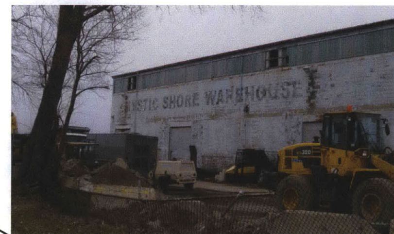
Abandoned-looking Atlantic Shore Warehouse as closest neighbor.
