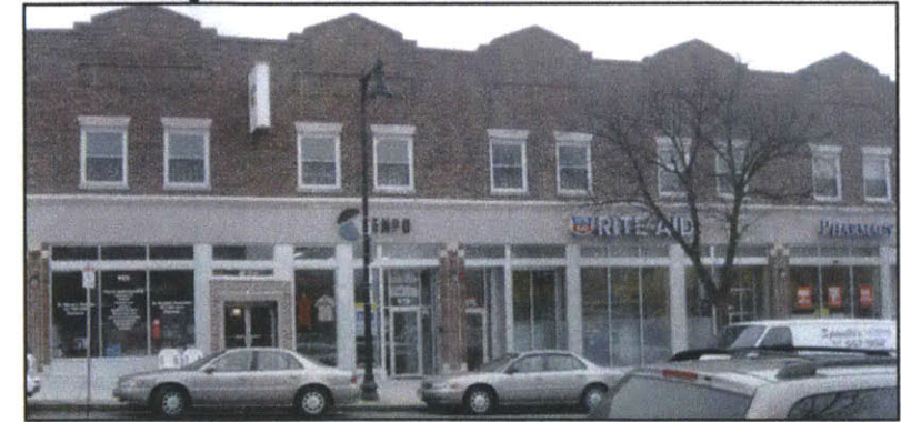
A multi-unit brick building with newer facade treatment may, due to better construction, last longer than other buildings on the street.
