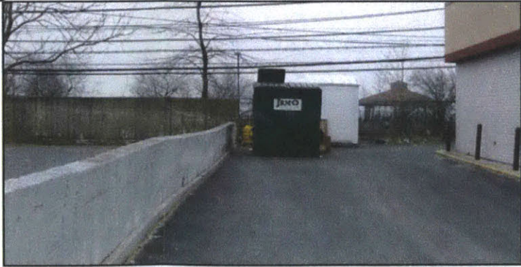
A restaurant may be protected from coastal floods by the concrete wall built around the back and sides of its property.
