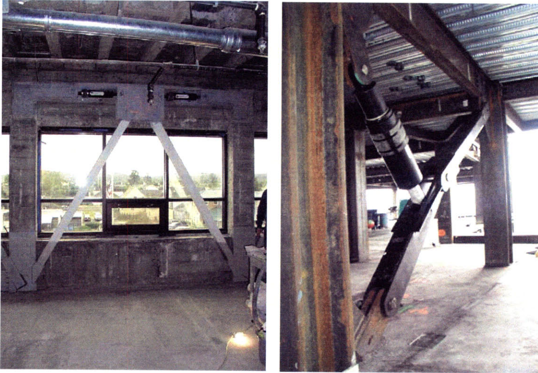
Figure 11:Viscous damper applications (Taylor, 2009)
