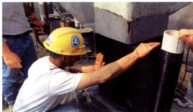
Figure 20: Retrofit of a RC column using a FRP jacket (Sps Repair, 2009)
