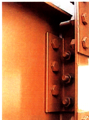
Figure 6: Internal-Type Accessory Connection – Bolts (adapted from Google Images)
