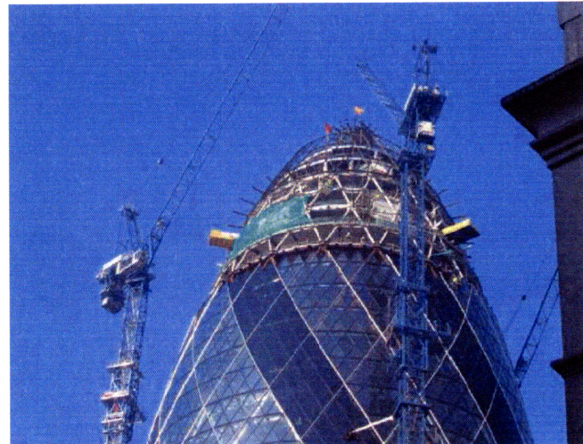
Figure 41 Image of Norman Foster's Swiss Re Tower under Construction [13]
