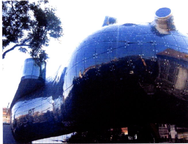
Figure 42 Image of Peter Cook's Graz Museum façade detail [8]
