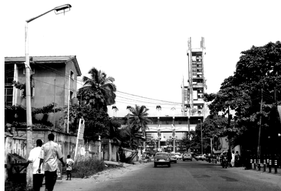
Vista to existing TBS
