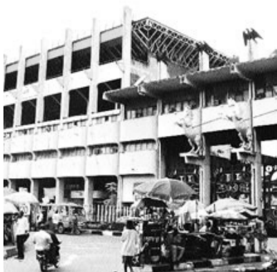
Existing TBS complex
