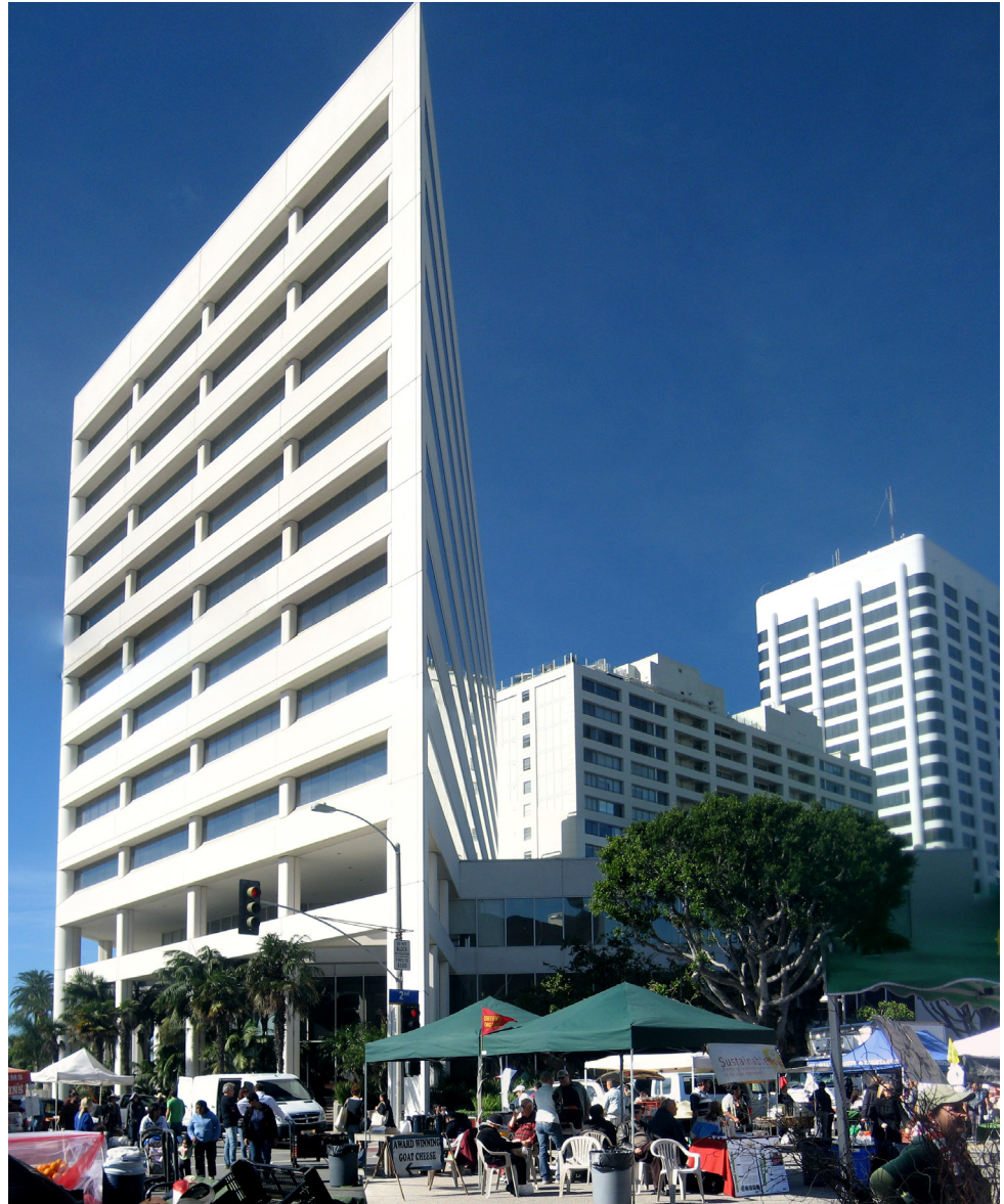
FIG 2.20: MARKET IN FOREGROUND OF ARIZONA AND 2ND STREET INTERSECTION
