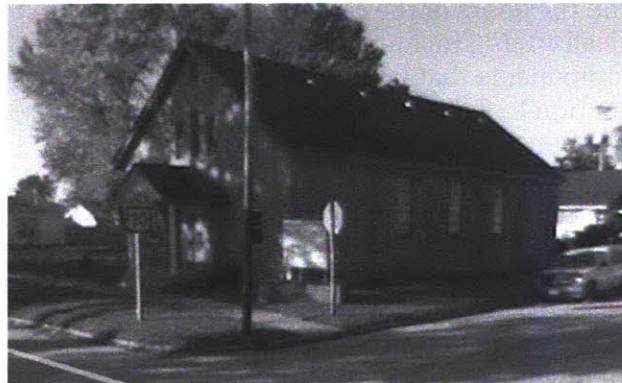
Figure 4. Grace Community Fellowship Church, built in 1954 (Google Maps).
