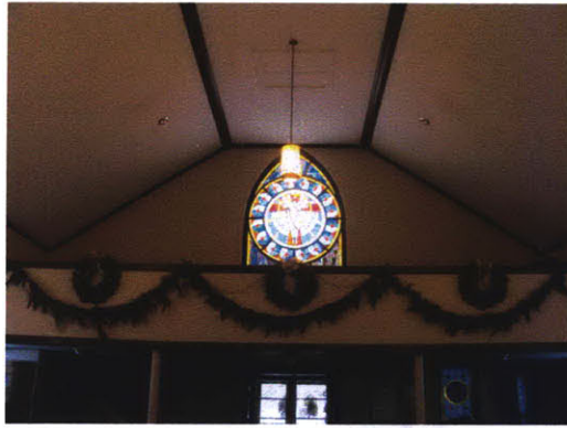
Figure 53. Dropped ceiling in St. Anne's Catholic Church in Logan, Iowa.
