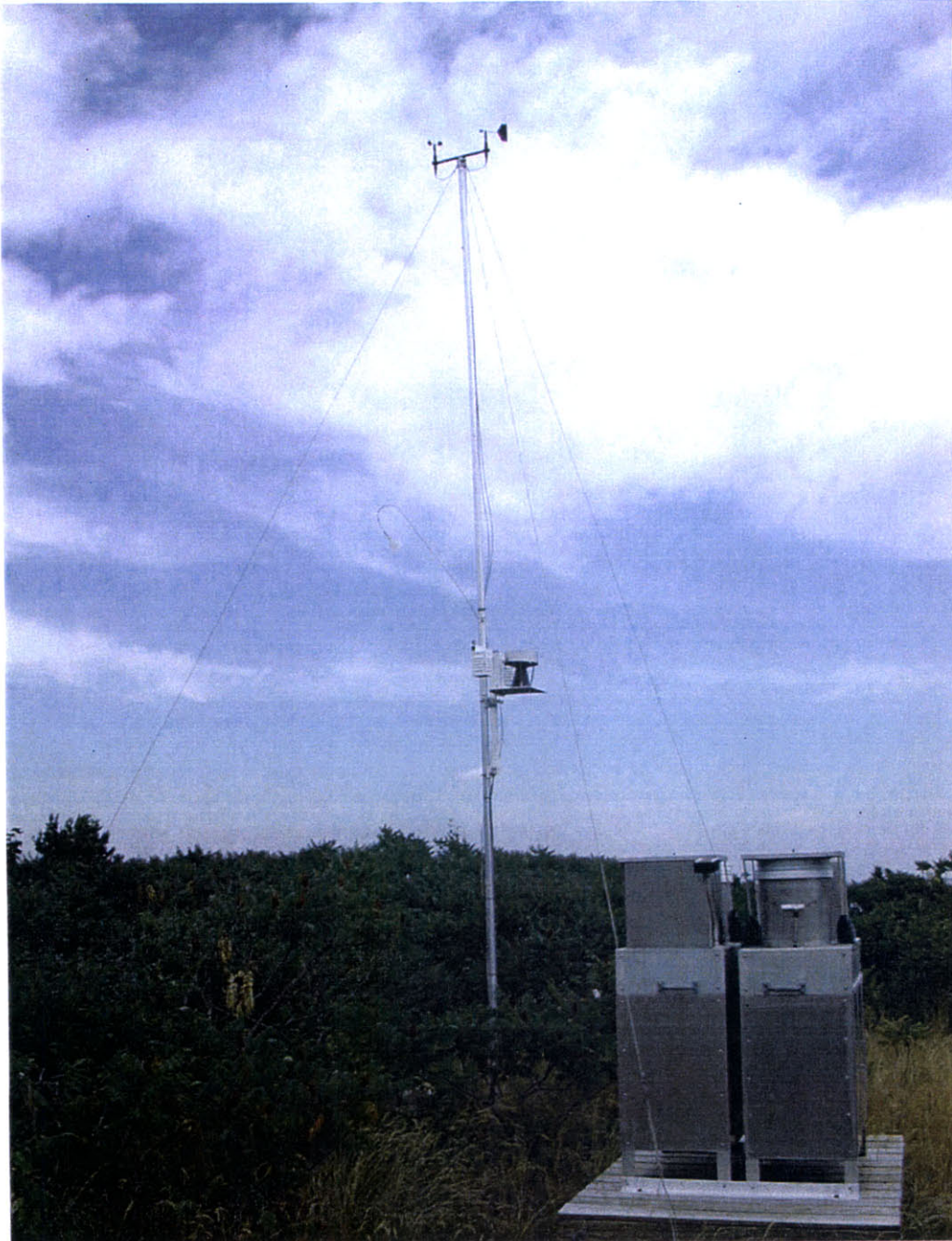
Air inlet on the roof of the bunker. 1/4" stainless steel tubing extends from the laboratory up through a ventilation shaft to this meteorological instrument tower. Our air inlet can be seen extending out to the left just over halfway up the tower. A teflon funnel is inverted at the end of the stainless steel tube to prevent water from being sucked into the tube.
