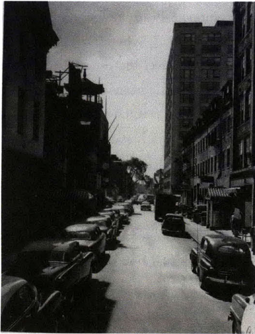
Source: To, Wing Kai and CHSNE Hudson Street, 1953 This photo was taken prior to the demolition of Hudson. The Eastern side was torn down to build an entrance ramp for the Turnpike.
