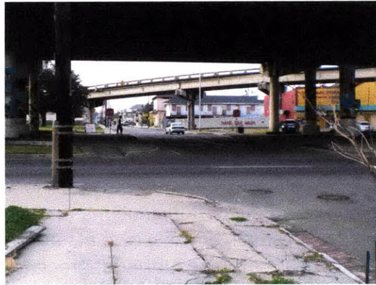
Figure 2.33 View across from under the bridge. Author's own image.
