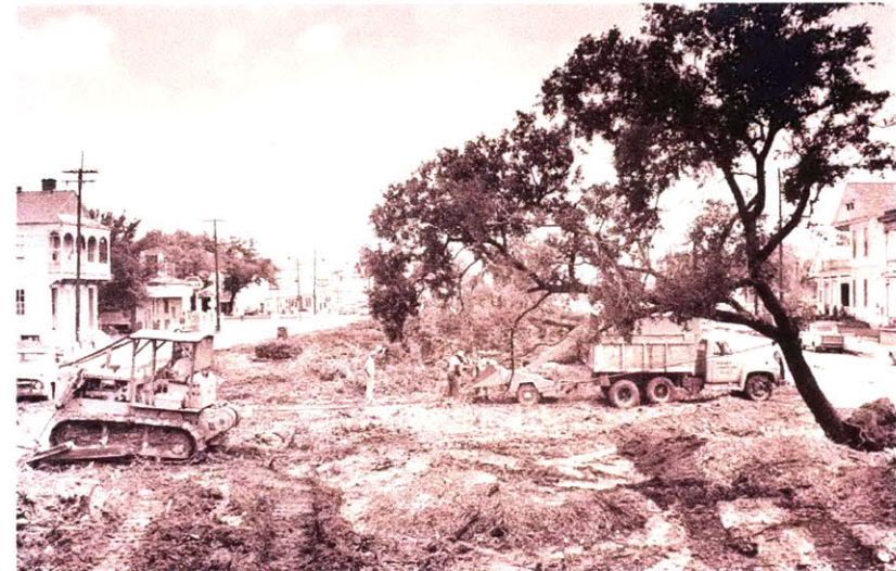
Figure 2.12: North Claiborne Avenue as removal of the oak trees begins in 1966. Source: Courtesy of William Borah
