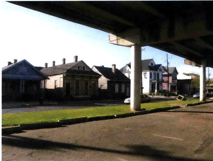
Figure 2.16: Homes along North Claiborne face the concrete roadbed.
