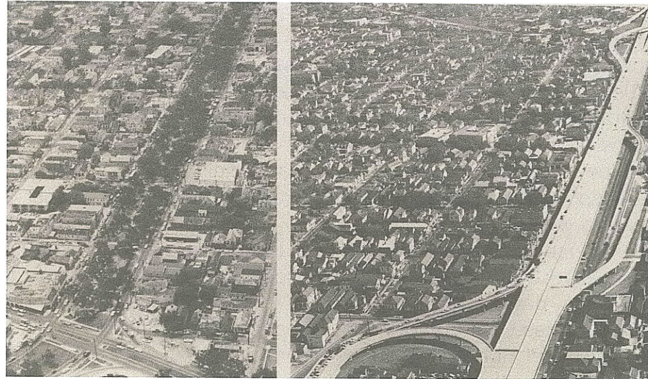
Figure 2.30 Aerials of North Claiborne Avenue before and after construction of the Claiborne Expressway. Source: CADT Study, 1976
