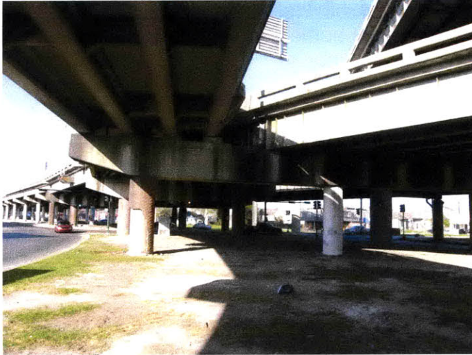
Figure 2.15: The Claiborne Expressway today.
