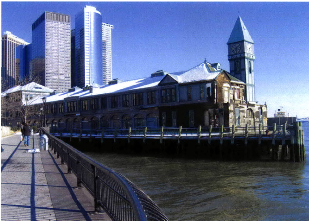
Figure 4.3 Current View of Pier A
