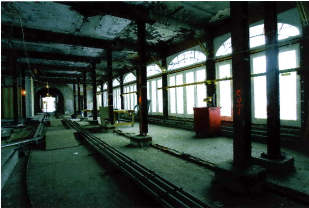
Figure 4.1 Interior View of First Floor
