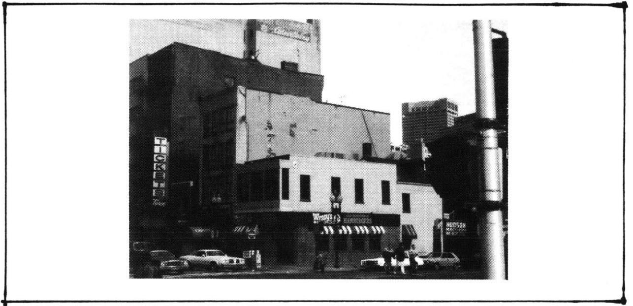
Southwest corner of "hinge block"
