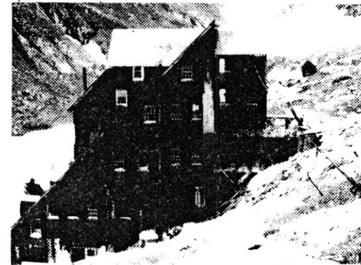
An Early Mine Building
