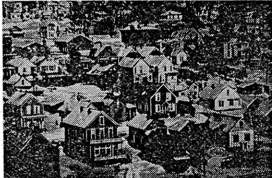
Typical fram buildings in the Historic Core
