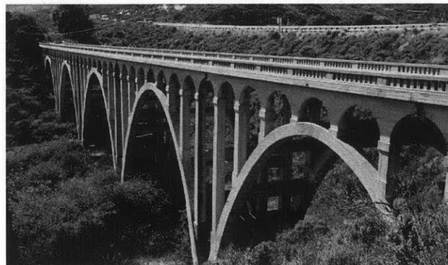
Figure 15 : Arroyo Quemado Arch Bridge
