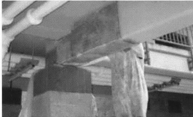
Figure 9 : Beam shear retrofitting of Challenger Middle School (Source : QuakeWrap)
