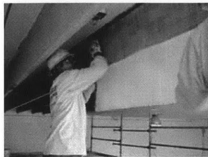
Figure 8 : Beam flexural upgrading of Oran Roberts Elementary School (Source : QuakeWrap)
