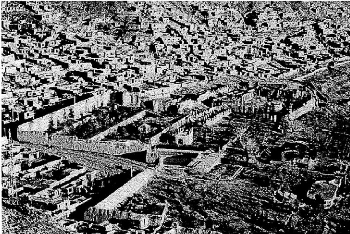
Elevated view of upper terraces from northwest, showing extent of damage prior to restoration, 1994. Source: Jolyon Leslie, Aga Khan Trust for Culture at www.archnet.org
