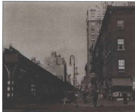
B. 1940. Automobiles, the elevated railway and pedestrians all share street space. Source: NYPL Digital Collection.
