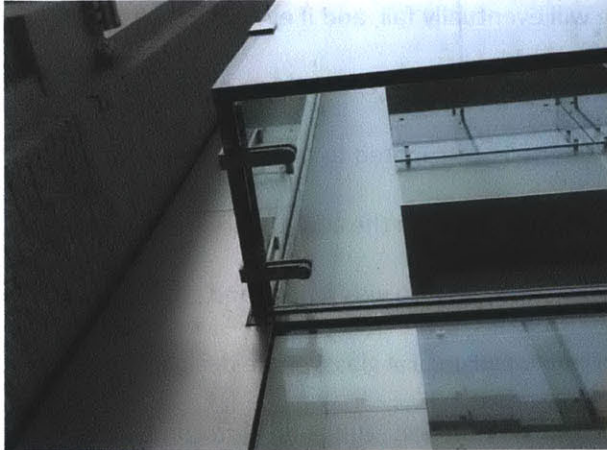
Picture 3: Exterior Façade Connection, Boston MA
