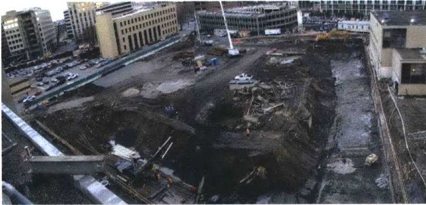
Photo of excavation progress on 11/28/2000
