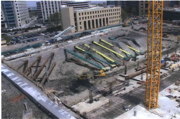
Photo of excavation progress on 5/04/2001
