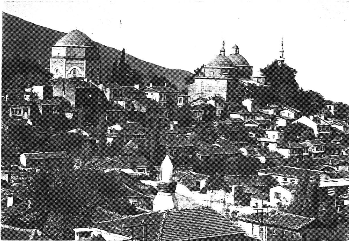
Figure 2.4 View of the kulliye at Yesil neighborhood; building at left is the tomb and to its right is the mosque
