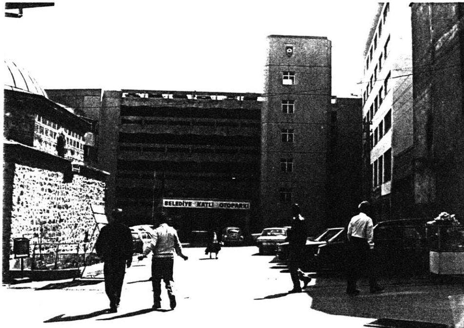
Figure 3.41 View of a multi-storey car park with a mosque adjacent to it
