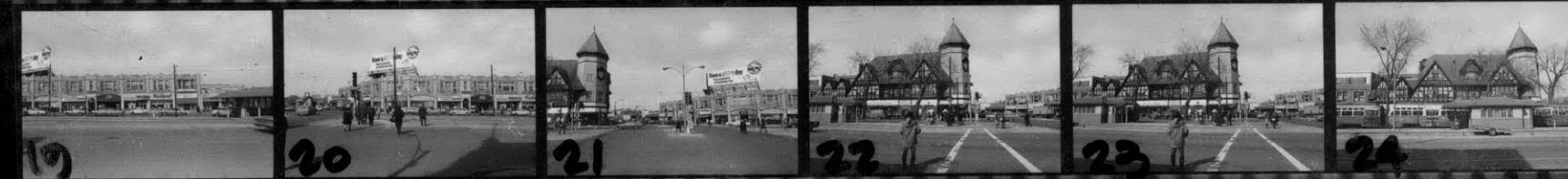
19 20 21 22 23 24 16-33 NORTHERN SIDE - BEACON ST.
