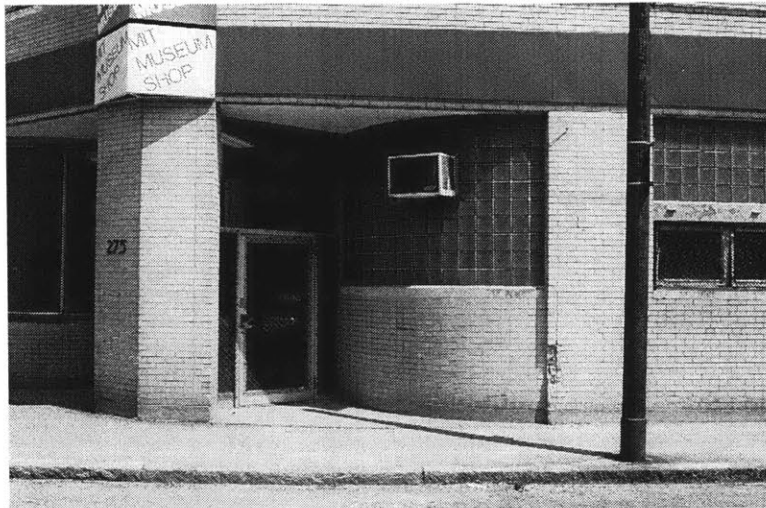
Fig. 14 Office N51-113 exterior view
